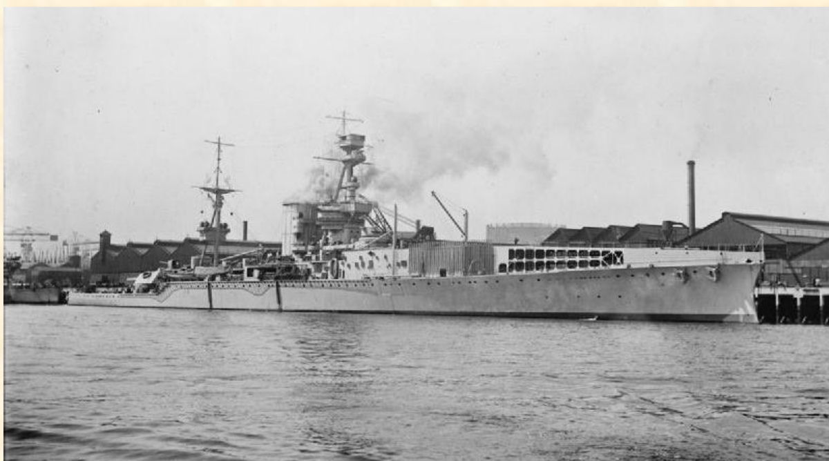
HMS Furious as originally completed in June 1917 by Armstrong Whitworth at their High Walker shipyard, just upstream from Jarrow. Note the flight deck forward of her bridge. Charles Clifford was a member of her first ship's company. (Surgeon Parkes Collection, Imperial War Museum, SP89 )
